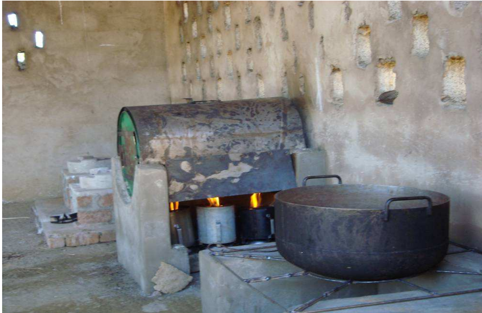
Bakery oven and big saucepan cooker (under construction) at Kasisi 2009.
