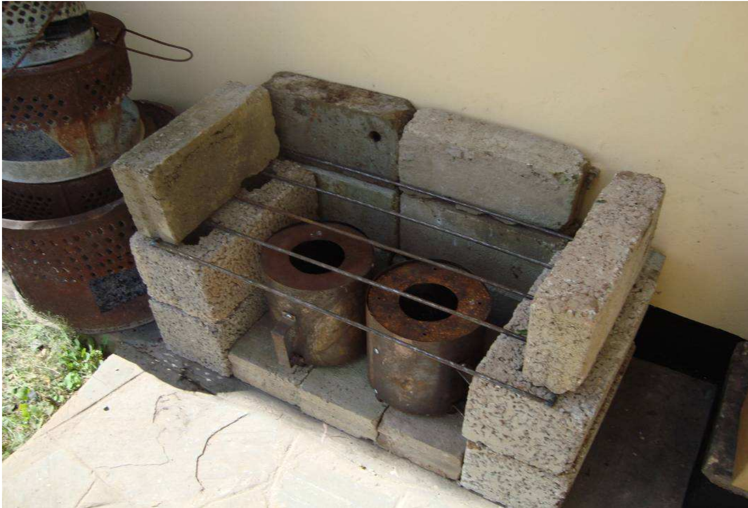
A cooking stand for two Peko Pe Units under construction.
