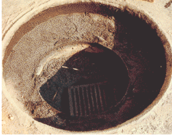
a) Interior structure of the combustion chamber
