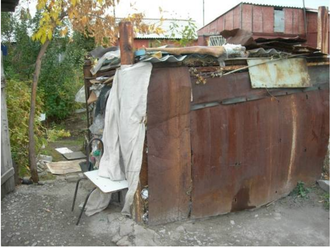
This is her heating supply for the winter.
