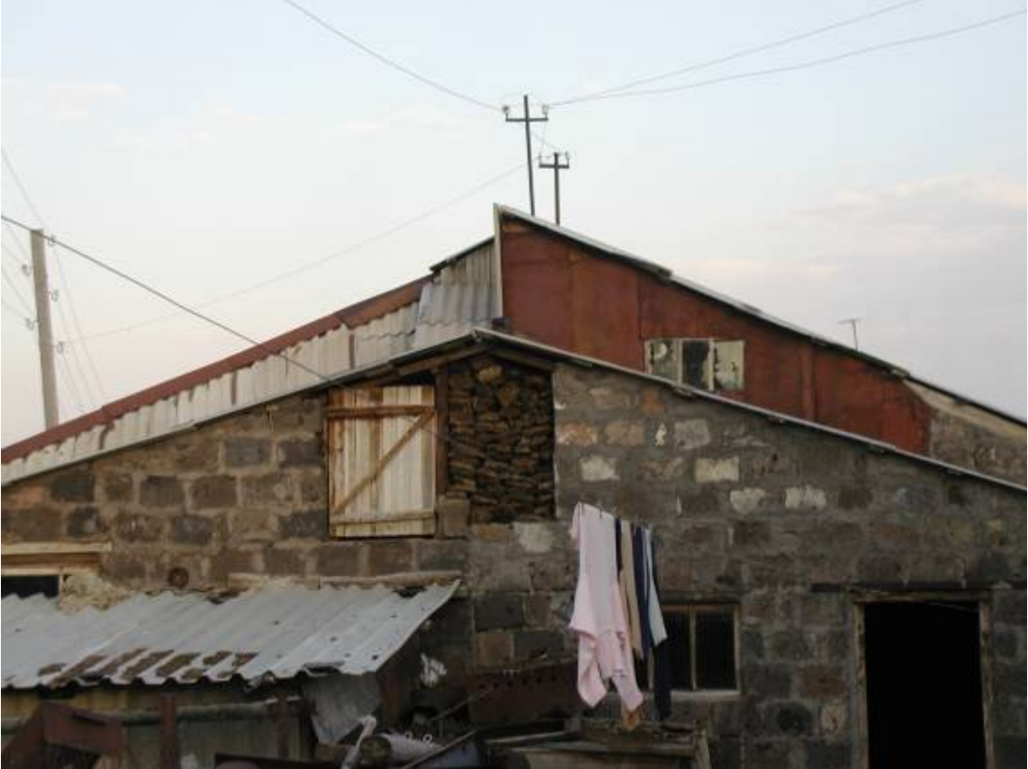
Manure being stored in the attic also serves as insulation.
