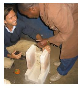
These bricks were then delivered in mid-July and were installed in the 2 mud stoves, the 2 modified WFP stoves, the 2 pot restaurant stove and the Satemwa Tea Estate 110L. The remaining bricks were used to fulfill the first WFP order for 55 stoves. The bricks form the 'L' shaped rocket combustion chamber (see photo left for partially built combustion chamber).
