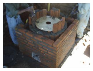
This stove was built for Satemwa Tea Estates in Thyolo. This stove is slightly different than the 100L EP stove as it was designed to fit the common 110L half drum, not the custom built 100L stainless steel pot. Wherever possible, we should discourage the use of these drums and encourage the use of stainless steel pots.
