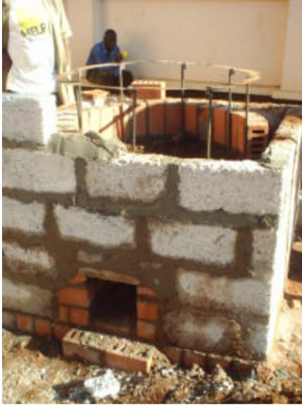
All Brick institutional stoves should now be built with this internal steel skeleton. This structure supports the pot, maintains the proper 15 mm gap between the pot and the stove body, and decreases stress on the brick stove body
