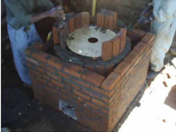
This stove was built for Satemwa Tea Estates in Thyolo. This stove is slightly different than the 100L EP stove as it was designed to fit the common 110L half drum, not the custom built 100L stainless steel pot. Wherever possible, we should discourage the use of these drums and encourage the use of stainless steel pots.
